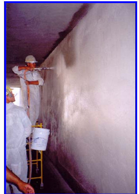
Placement of the Reinforcing Mesh HD and spray application of Cem-Kote Flex Plus
