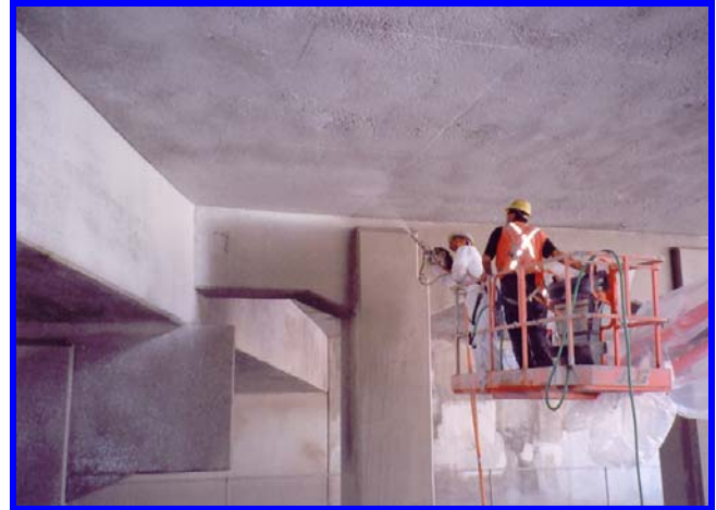
Spray application of Cem-Kote Flex Plus
