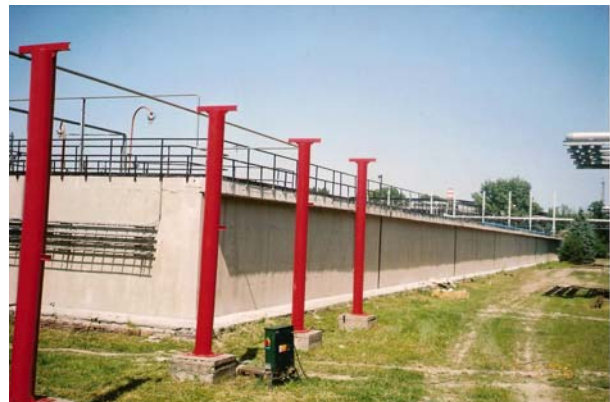
Figure 18. Exterior of the tank after the repair
