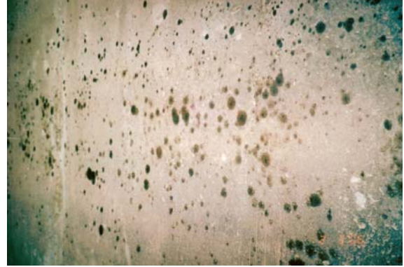
Figure 8. Residual emulsified oil “seeping out” of capillaries after sandblasting and high-pressure wash
