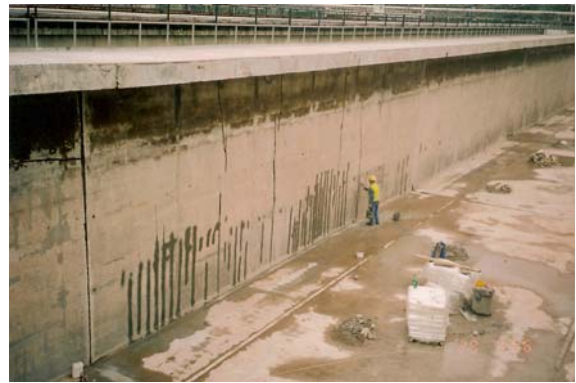
Figure 12. Delamination repairs using fibre reinforced mortar and polymer cement rust-proofing .
