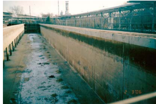
Figure 6: The surface of the tanks after chemical cleaning
