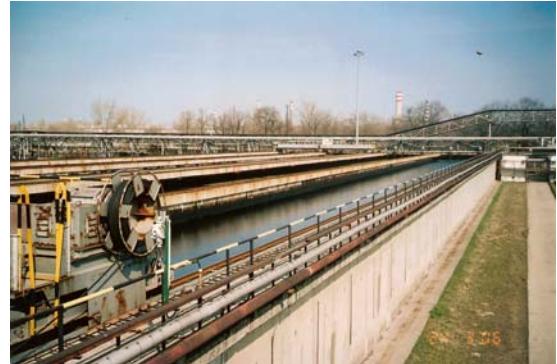
Figure 2. The second tank before the repair
