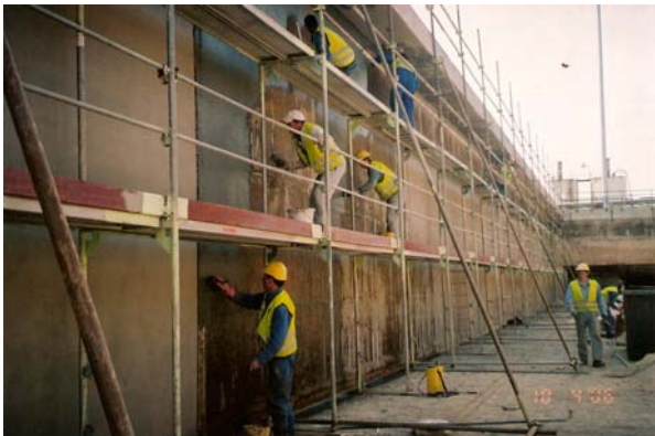
Figure 15. Application of the bonding agent and protective/waterproofing coating.
