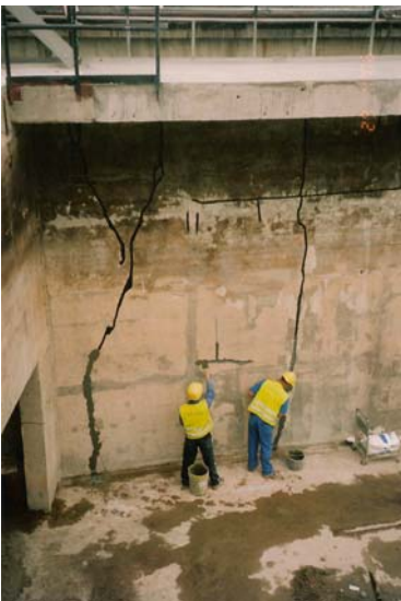
Figure 9. Filling the routed cracks with one component polyurethane
