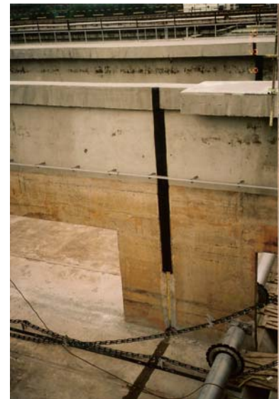
Figure 14. Repair of the vertical expansion joint.
