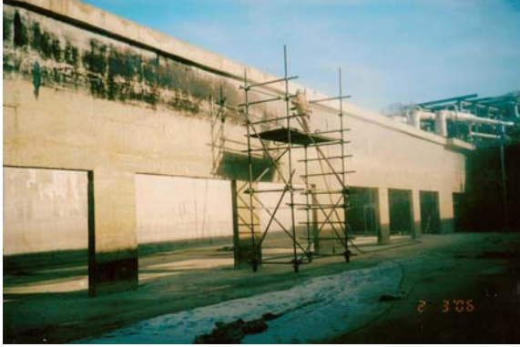
Figure 7. Sandblasting after chemical cleaning
