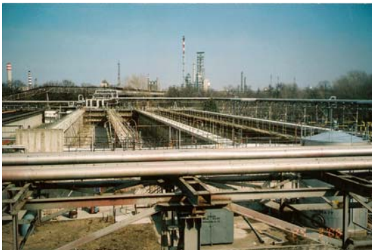
Figure 1. The first tank during the repair
